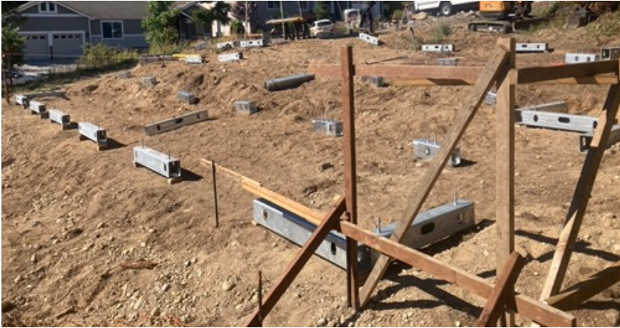
Sloped lot with Ground Frame Beams
