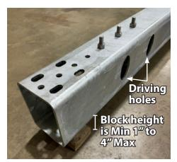
**5.** Block and shim the end of the steel beams to the same level as the master corner or within leveling plate adjustability range. Minimum block height is 1" and maximum height is 4" for frost heave. Ensure driving holes remain open and are not blocked by shims.
