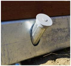
**16.** Install pipe caps on top of each pipe.
