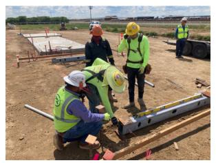
**6.** Verify all outer dimension according to the dimentioned layout. Ensure steel beams are plumb, level, and square to the overall layout.
