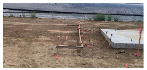
**1.** Using the dimensioned layout as a guide, establish the container border with a string line. Ensure alignment with string line.
