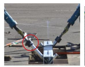
**13.** Stop driving prior to bit hitting the beam.
