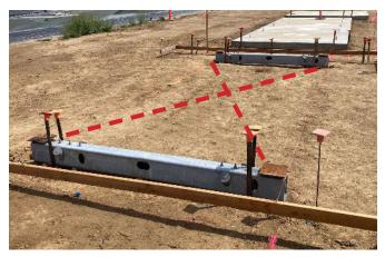
**3.** Measure diagonally to ensure the border is squared.
