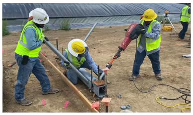
**12.** While holding the pipe up, drive the pipe through the side driving hole, using the jackhammer with the pipe driving bit.
