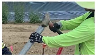
1. Using a sledgehammer, strike the pipe, 3-5 blows, to ensure pipe refusal.
