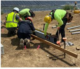
**7.** Upon leveling completion, gather and stage Ground Frame pipes.
