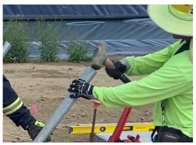
**10.** Using a sledgehammer, drive the pipe in a few inches, to maintain the proper angle.
