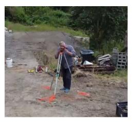
**4.** Find the elevation of a "Master Corner" (the highest corner).
