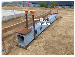
Best practice is to cradle the beam with 4 stakes to ensure it stays on layout when driving pipes. Continue to page 7 for pipe installation.
