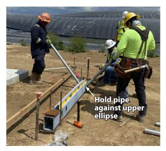
**9.** To ensure the pipe maintains the proper angle, hold it against the upper ellipse of the side driving hole.
