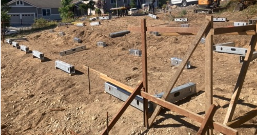
Sloped lot with Ground Frame Beams
