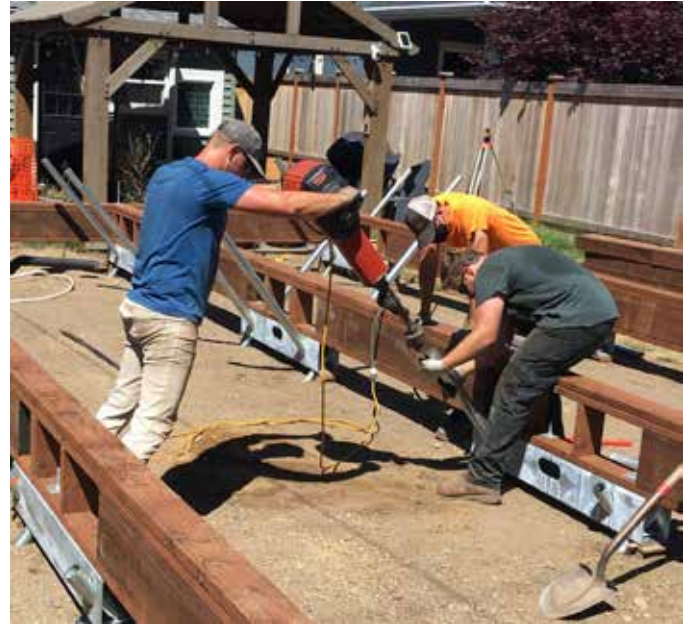
Backyard DADU under construction in Tacoma, WA
