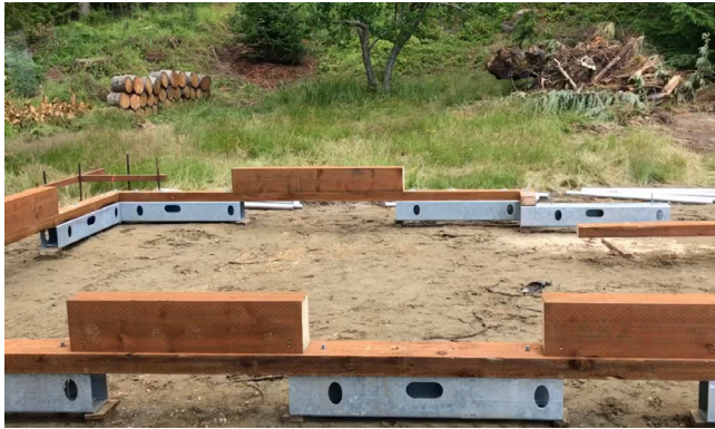
15. Continue installing the sill plates and headers.
