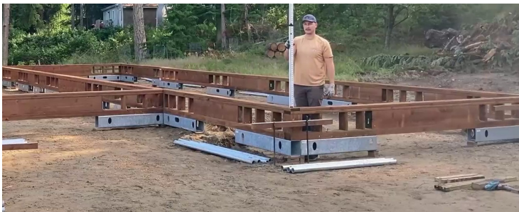
17. Double check your elevations and make any necessary adjustments.
